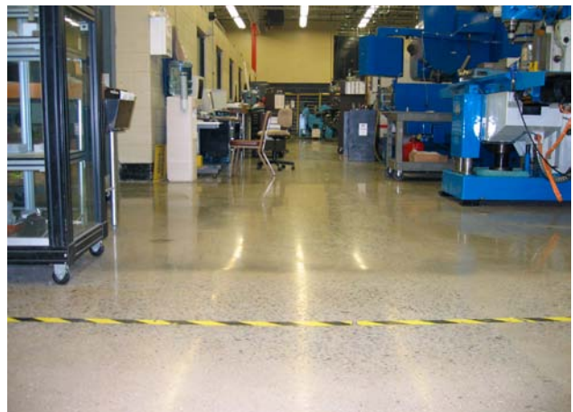
After removal of industrial epoxy coatings & polished to HTC Superfloor™ Platinum
