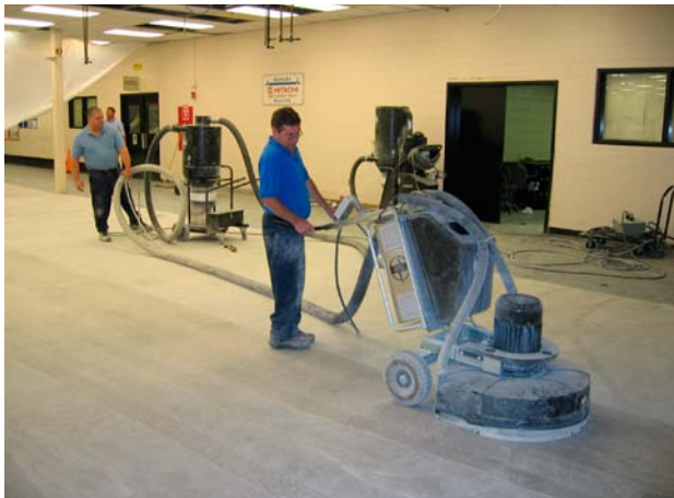
Keith Smith and Eric Stratton grinding and polishing their factory floor with the HTC 800 HD Classic
